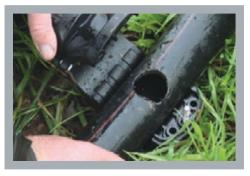
3. Ensure the internal seal is installed. Use the small white spigots to help locate it correctly. Place the Hansen Fast Fit Tapping Saddle around the pipe using the saddle spigot to help locate it in the drilled hole. Tighten bolt.
