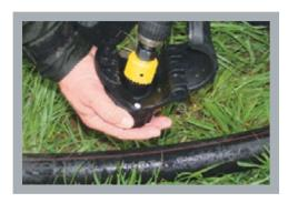
1. Select a hole saw to fit between the min. and max. as marked on the saddle body of your Hansen Fast Fit Tapping Saddle.
