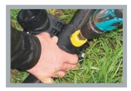
2. Use the pilot hole located on the base of the Hansen Fast Fit Tapping Saddle as a guide to start drilling, then remove the Hansen Fast Fit Tapping Saddle and complete the drilling. Clean off the burrs from the pipe.
