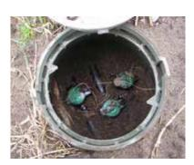
Where the soak hole option is chosen, the flush valves can be terminated in a chamber over the soakhole
