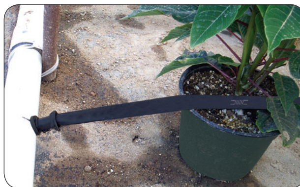
Figure 2: PVC pipe supply header with Space-It Dripline.
