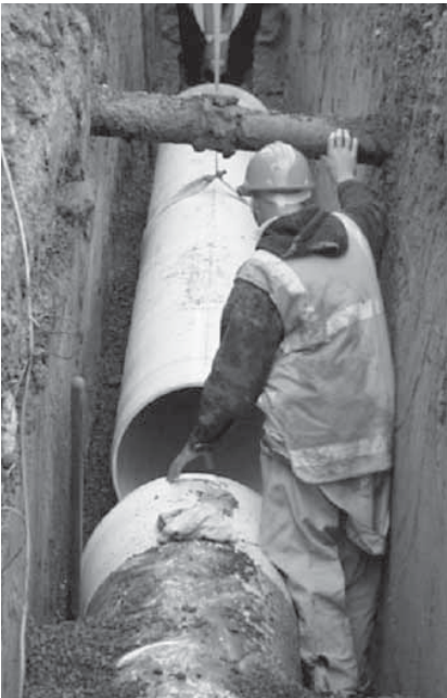
Installation of DN575 (630mm OD) PN9 White RHINO watermain under sealed road. NB: normally, trench shields would be required at trench depths greater than 1.5m.
