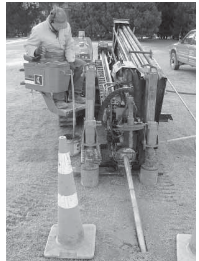
Assembly and installation of DN150 RESTRAIN gravity sewer, replacing an old EW sewer by pipe reaming with a horizontal directional drill.
