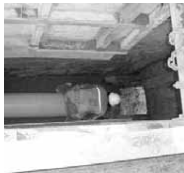
Deep installation of NOVADRAIN DN300 SN4 at 4.8m cover under main road.
