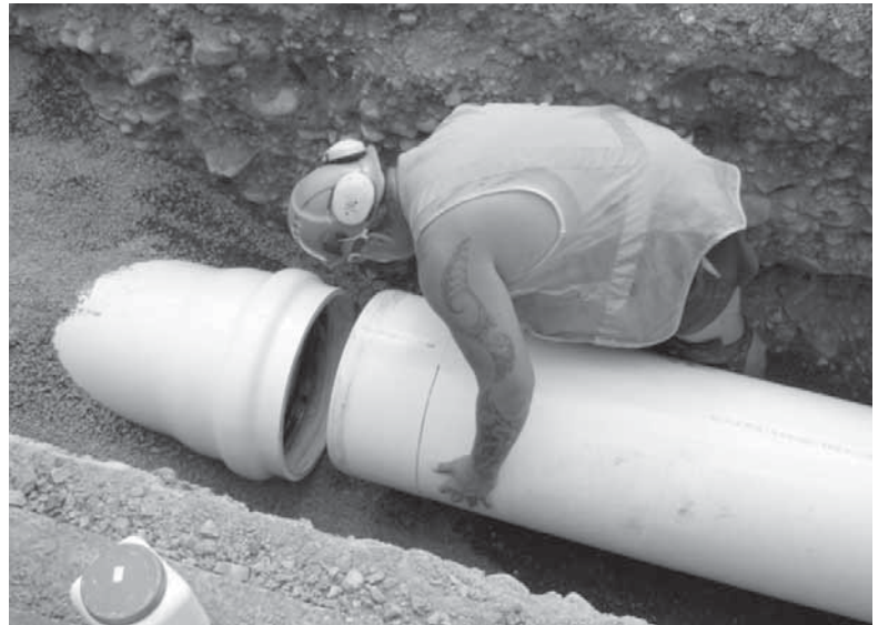
Joint assembly on NOVAKEY DN 450 PN12 watermain under a sealed main highway.
