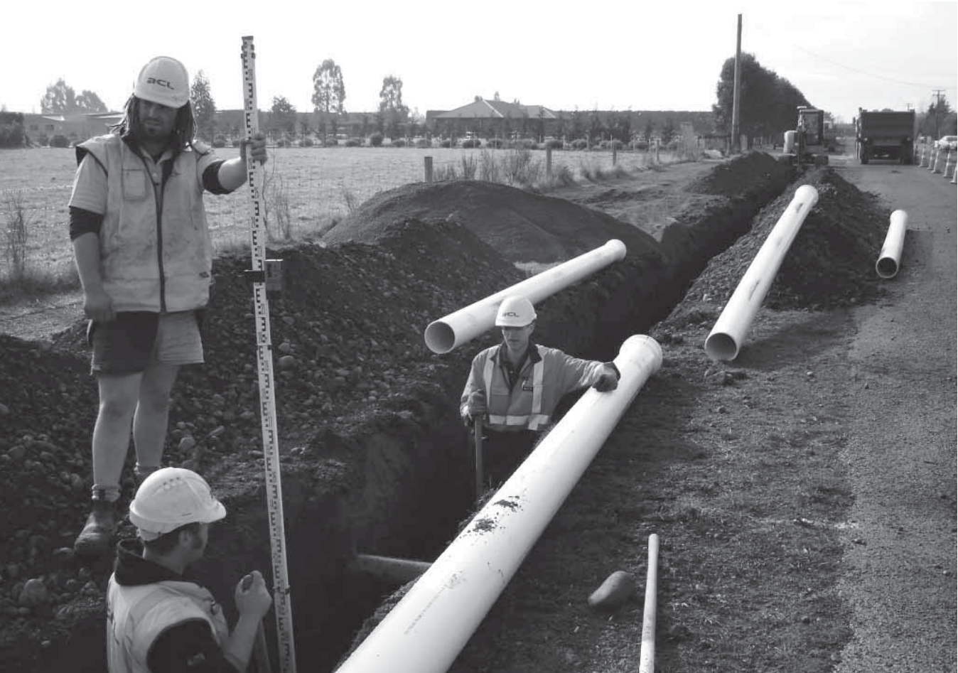
Installation of Novakey Series 1 PN 12 pipes, in a road berm, with laser assisted control of the trench depth and grade.
