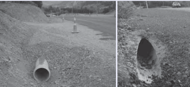
DN300 PVC-U stormwater pipe used as a road access culvert. (Left) Immediately after installation and (right) 18 months later, showing the effectiveness of well placed and thoroughly compacted bedding and surround aggregate material.
