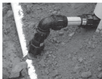
BlueLine pipe and Plasson compression fittings used for a water service connection to a residential property.
