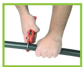
1 Cut the pipe with pipe cutters, a knife or saw. Ensure a square cut of pipe ends. Clean burs off pipe. When making a repair in a burst pipe make sure the length of the cut away matches the length of the replacement fitting between the screwed on nuts.
