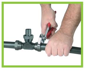
**3** Wind the nut onto the pipe a few turns. Tighten with spanner or pipe grips.
